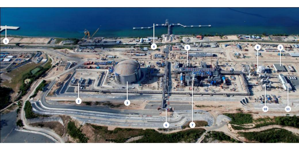
Material Offloading Facility 2. Refrigerant Storage 3. LNG Tank 4. LNG Jetty 5. Air Fin Coolers 6. Flare 7. MCHE
