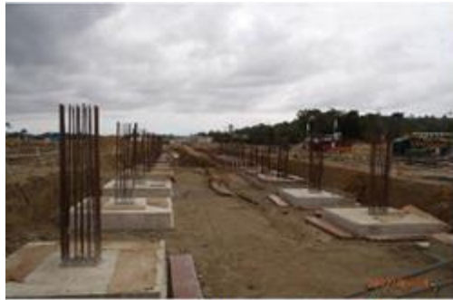
E130 : Admin Building Area - Foundation Work, Rebar & Form Works.
