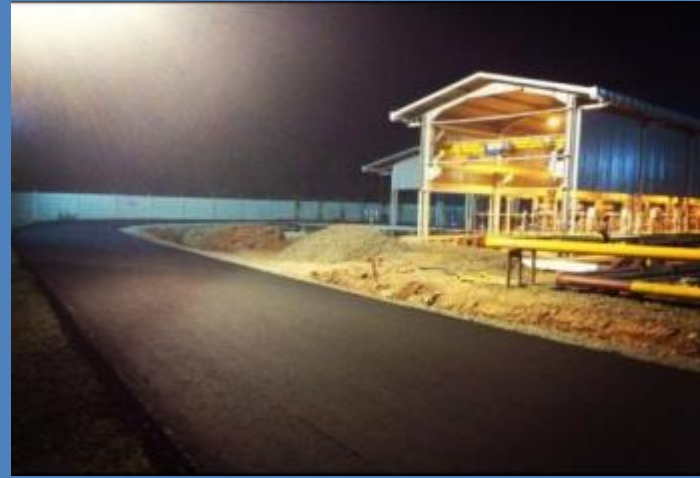
Asphalting Road (Eastern Side)
