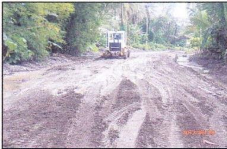
Fixing access road from Senoro 1 to Quarry 2
