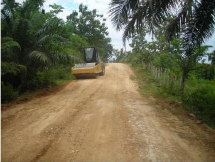
Compaction access road to Matang-1 well site
