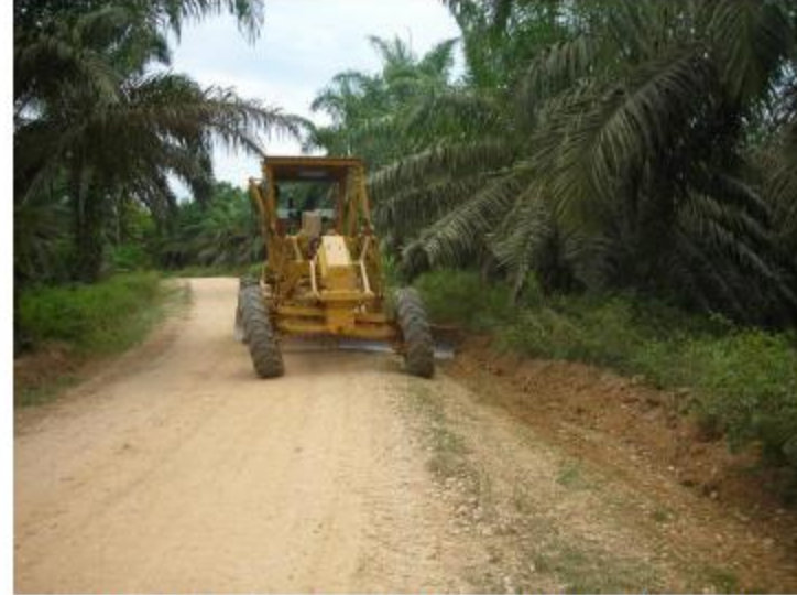
Grading access road to well site location
