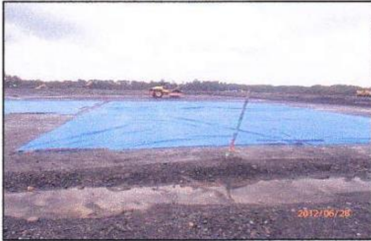
Laying out tarp in the CPP Area
