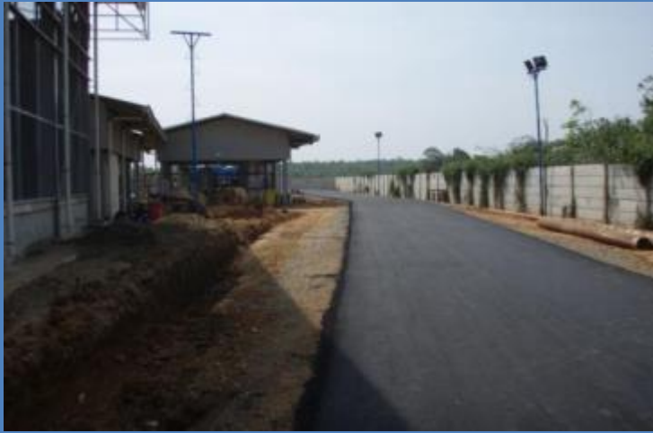
Asphalting Road (Northern Side)
