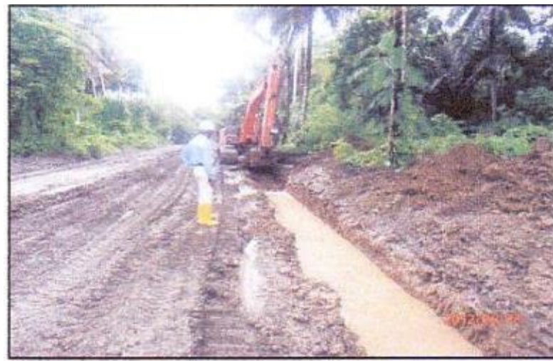
Drainage construction in access road from Senoro 1 to Quarry 2
