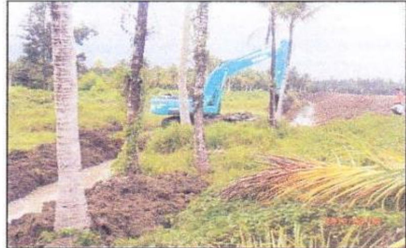
Clearing alternative access road to CPP area
