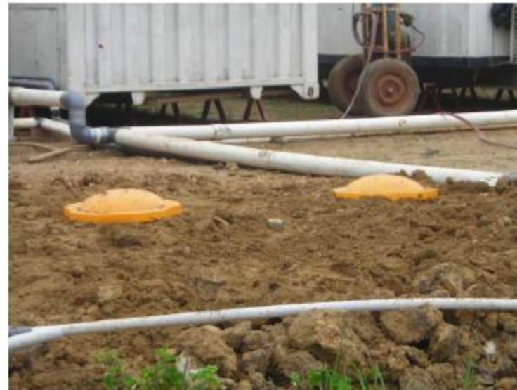
Back fill wastewater disposal tank
