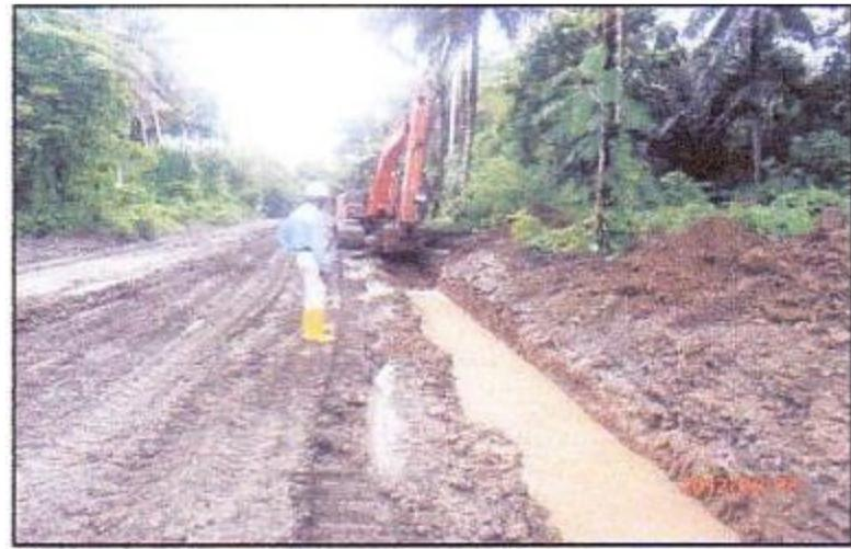
Drainage construction in access road from Senoro 1 to Quarry 2
