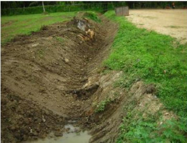
Excavation drainage at Site Camp
