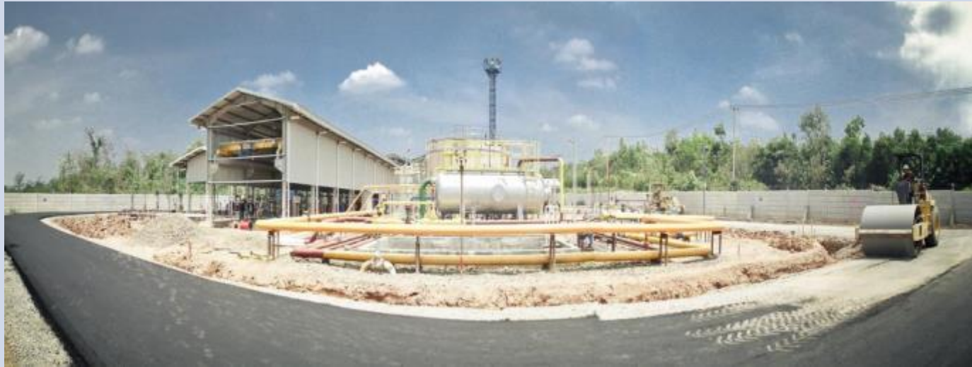
Road Asphalting on EOR Pilot Area
