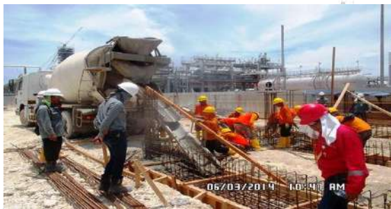
Control Room Building
