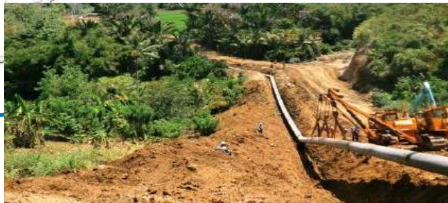
Lowering at KP 10+000
