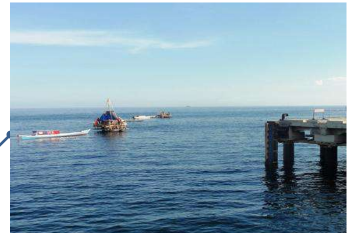
Soil Investigation (BH-05)
