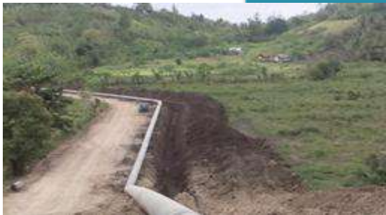
Trenching Pipeline
