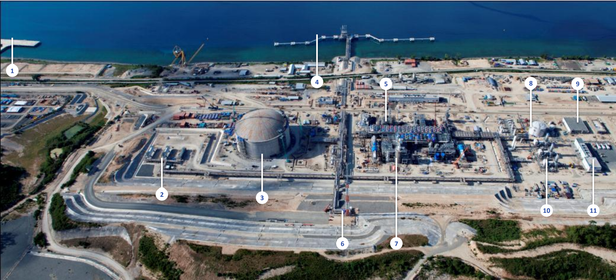
1. Material Offloading Facility 2. Refrigerant Storage 3. LNG Tank 4. LNG Jetty 5. Air Fin Coolers 6. Flare 7. MCHE 8. Firewater Tank 9. Main Control Room 10. Gas Turbine Generators 11. Main Substation
