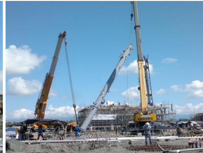
Erection Amine absorber
