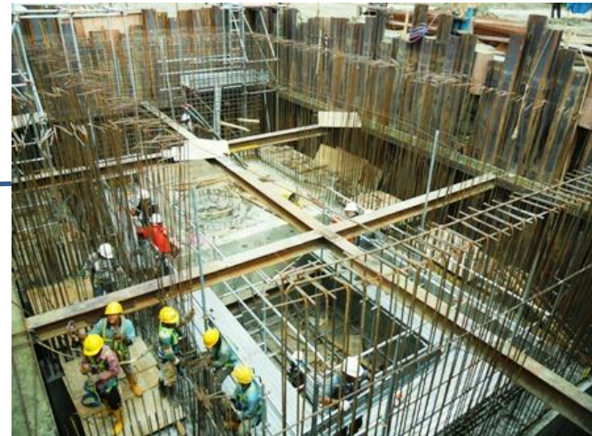
Pit Pond #11 Shoring
