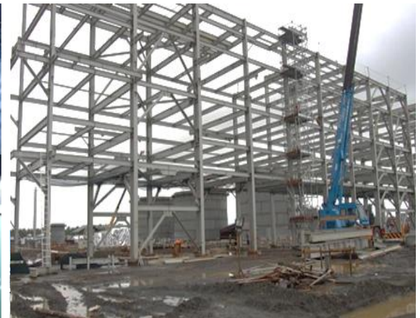
Main Pipe rack
