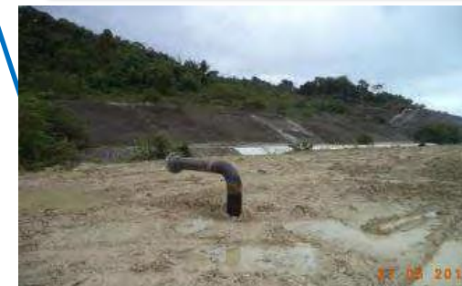
Backfilling at KP 22+000
