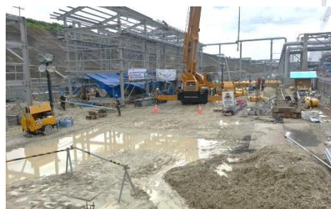
Shelter Gas Custody Transfer Metering Package, Erection
