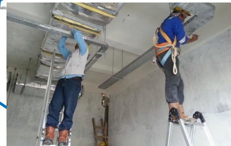
Control Room, Cable Tray Installation
