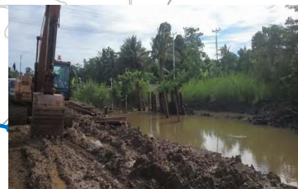
Pipeline Works at KP 4+500
