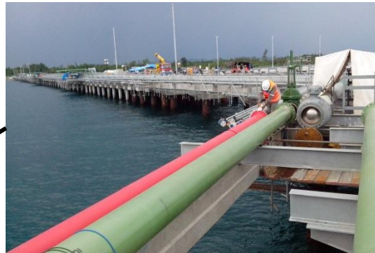
Blowing Utility Line
