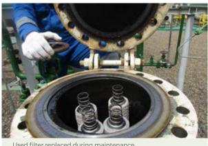
Used filter replaced during maintenance
