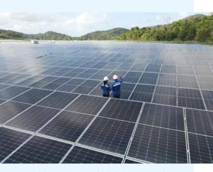
Indonesia is blessed with ample irradiation for Solar PV, particularly in Nusa Tenggara and Bali. Medco Power has developed and now operates the largest land-based solar PV power plant in the country, the 26 MWp Sumbawa solar PV. It replaces the diesel facility of the AMNT mine with a CO<sub>2</sub> reduction of nearly 40,000 ton/annum.
