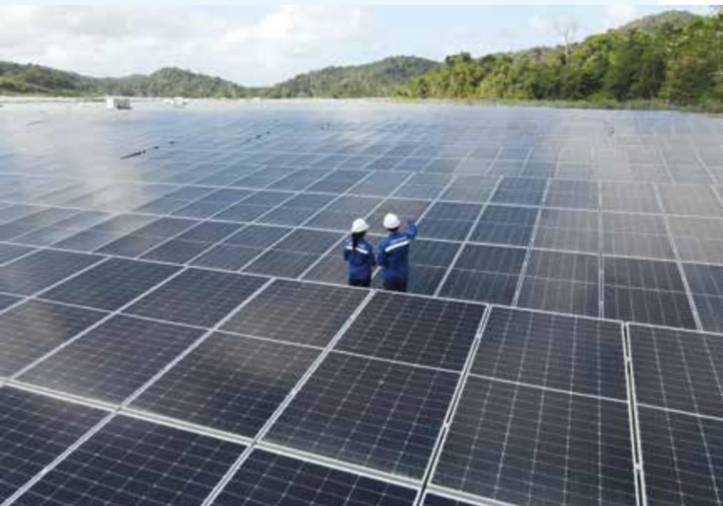
Indonesia is blessed with ample irradiation for Solar PV, particularly in Nusa Tenggara and Bali. Medco Power has developed and now operates the largest land-based solar PV power plant in the country, the 26 MWp Sumbawa solar PV. It replaces the diesel facility of the AMNT mine with a CO<sub>2</sub> reduction of nearly 40,000 ton/annum.
