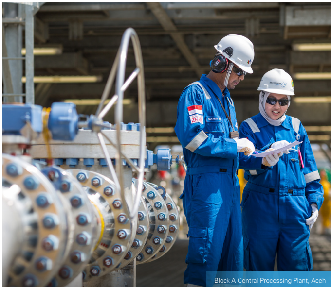
Block A Central Processing Plant, Aceh
